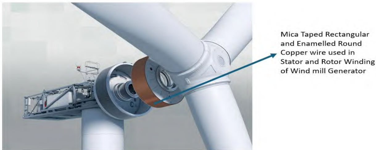
Figure 2: Use of Winding Wires in Turbine Generator
