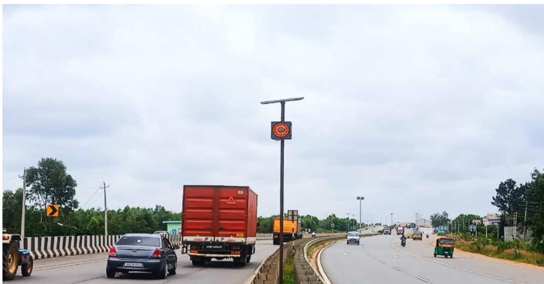
Figure 7.11: Photographs showing LED Blinkers
