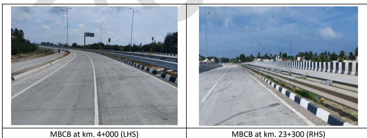
Figure 6.6: Photographs of W Beam Crash Barrier
