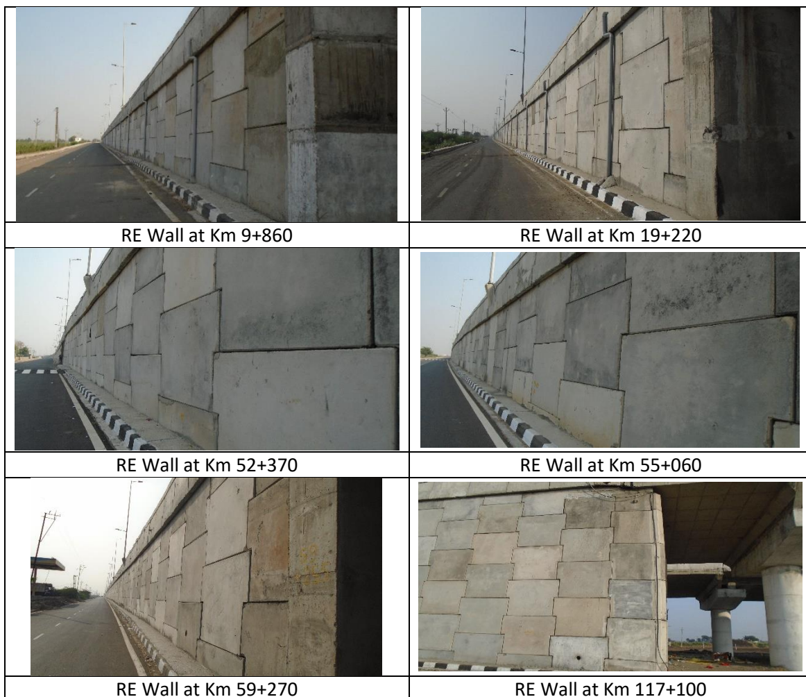
Figure.7.4: Photographs showing the status of RE Wall
