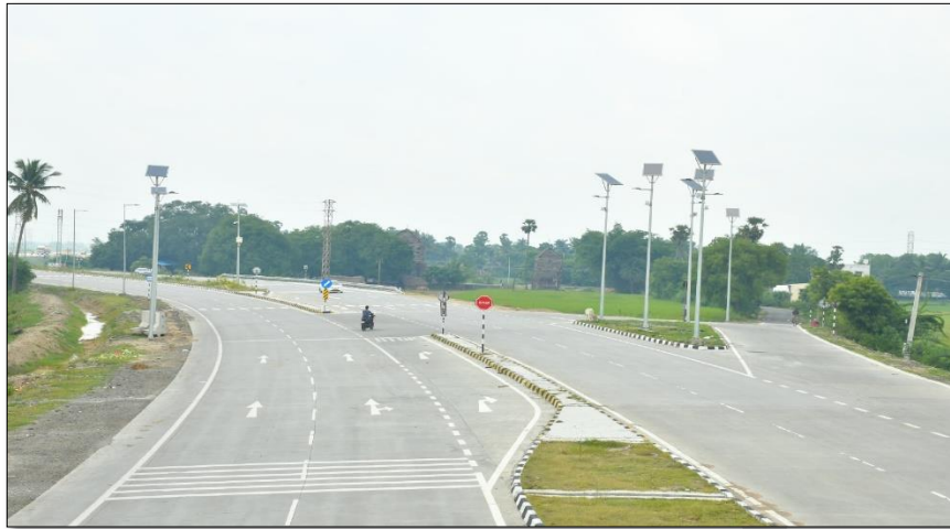
Ch: 1+580 median opening & junction area solar lights fixed
