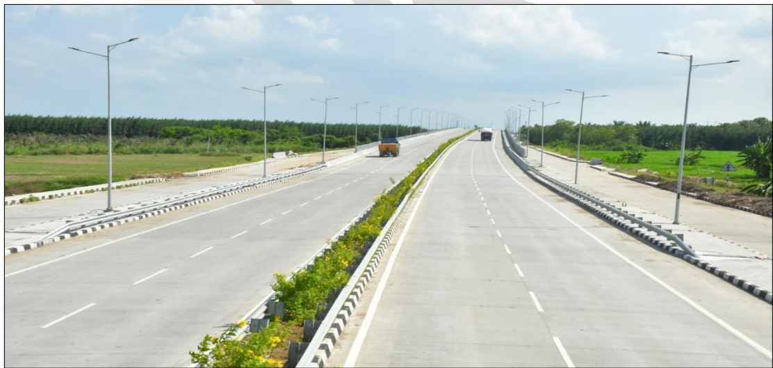
CH: 15+000 TO 15+500 MCW & SR MBCB, MEDIAN PLANTATION, RCC DRAIN & URBAN LIGHTS FIXED
