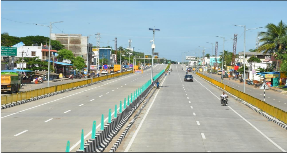
CH: 19+300 TO 20+000 MCW & SR NJCB WITH ANTI GLARED POST, GUARD RAIL, VASD, PTZ CAMERA, GANTRY BOARD, RCC DRAIN & URBAN LIGHTS FIXED
