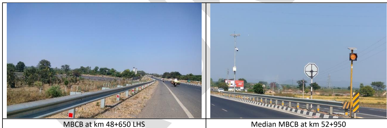
Figure 7.10: Photographs showing the Condition of MBCB
