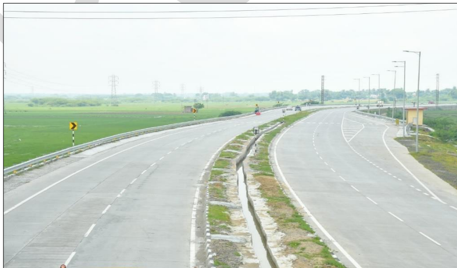
Ch: 2+100 to 2+350 Median Drain & Bus bay with Shulter, urban light fixed
