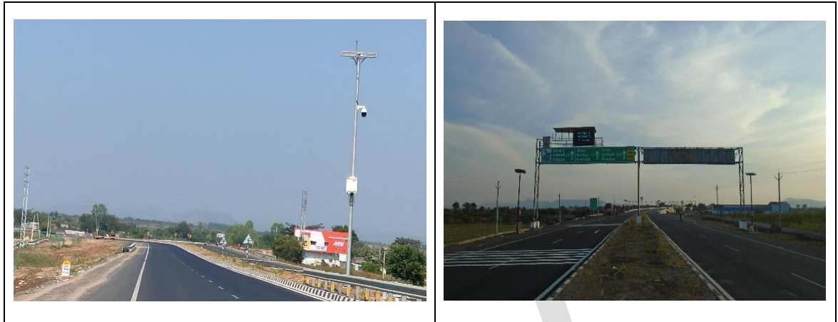
Figure 7.16: Photograph showing the VMS boards in the project road
