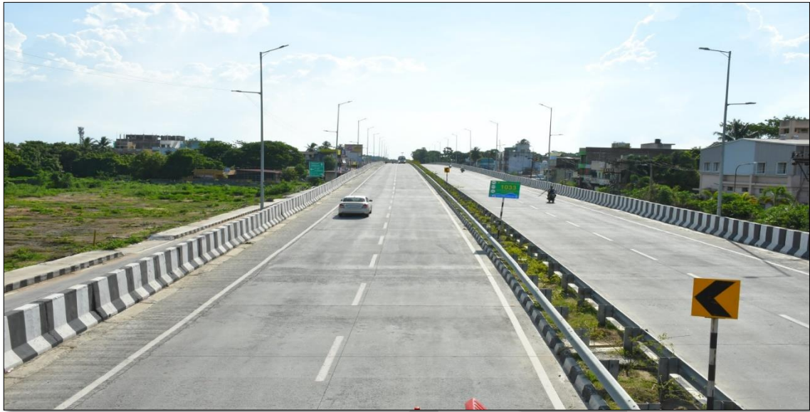
CH: 21+600 TO 21+900 VUP LOCATION, MCW & SR MBCB, MEDIAN PLANTATION, RCC DRAIN, URBAN LIGHTS FIXED
