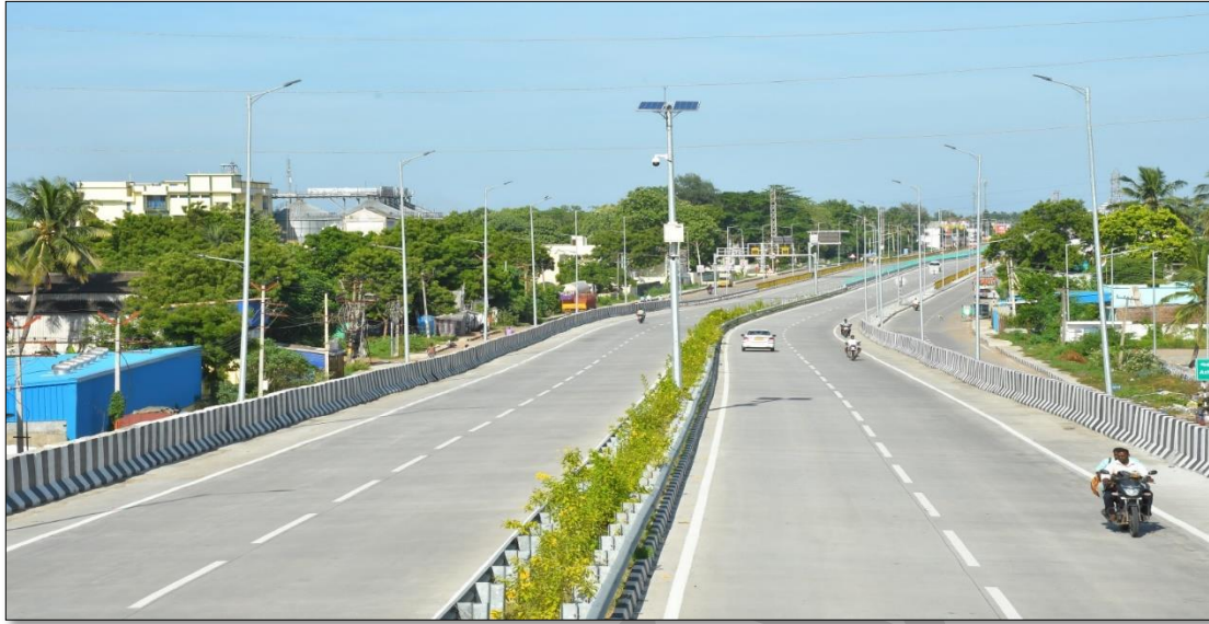
CH: 23+500 TO 24+000 MCW & SR MBCB WITH PLANTATION, NJCB WITH ANTI GLARED POST, GUARD RAIL, VASD, PTZ CAMERA, RCC DRAIN & URBAN LIGHTS FIXED
