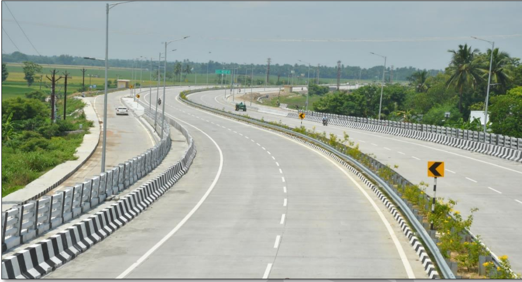
CH: 5+000 TO 5+200 MCW & SR CURVE LOCATION MBCB, MEDIAN PLANTATION, BUS SHULTER, RCC DRAIN & URBAN LIGHTS FIXED
