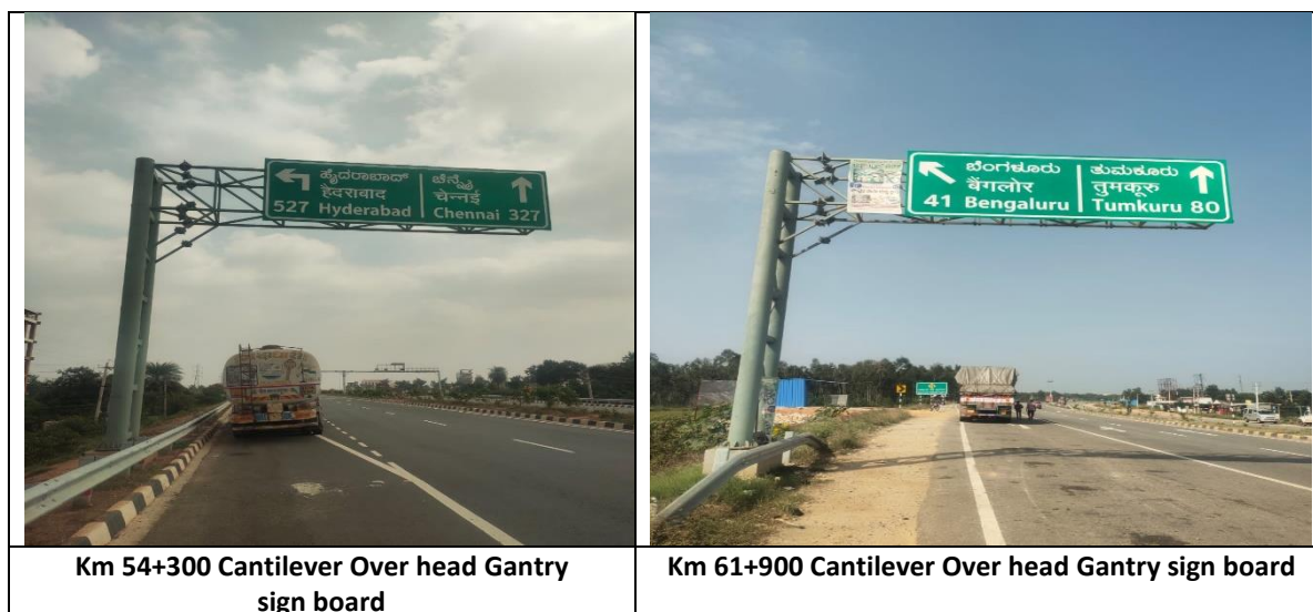
Figure 7.8: Photographs Gantry Sign Boards
