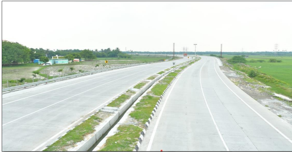
Ch: 2+600 to 3+050 Median drain in Super Elevation portion
