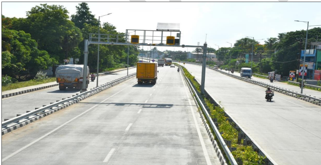
CH: 22+000 TO 22+300 MCW & SR MBCB WITH MEDIAN PLANTATION, VASD, RCC DRAIN & URBAN LIGHTS FIXED
