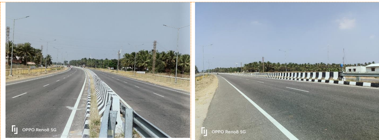
New Jersey Crash Barrier at Built up area location in the median, end termination connection with MBCB
