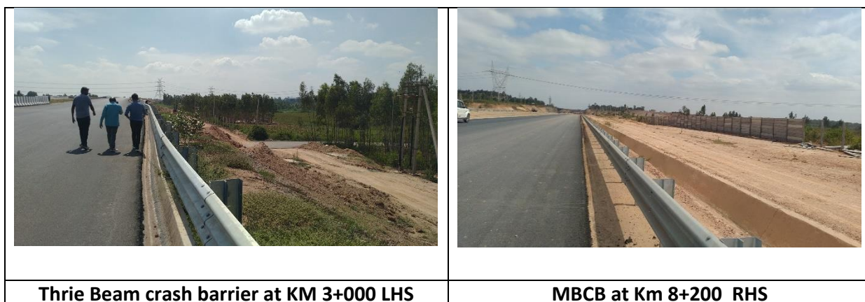
Figure 7.3: Photographs of Metal Beam Crash Barrier
