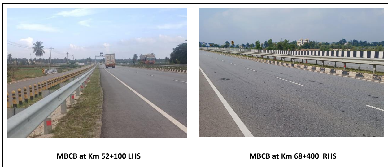
Figure 7.12: Photographs showing W Beam Crash Barrier
