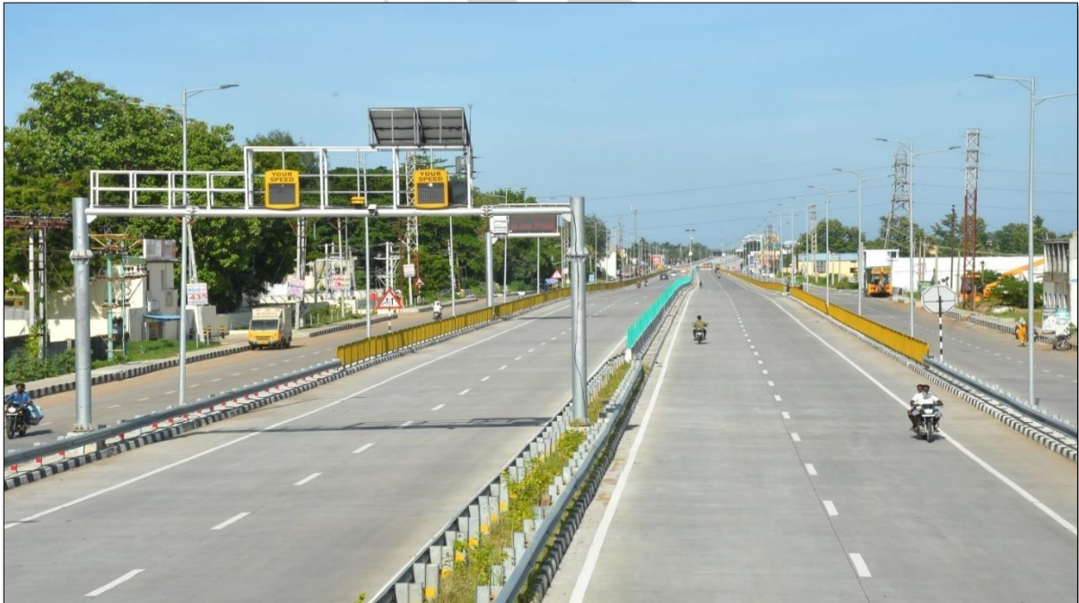
CH: 24+000 TO 24+900 MCW & SR MBCB WITH PLANTATION, NJCB WITH ANTI GLARED POST, GUARD RAIL, VASD, RCC DRAIN & URBAN LIGHTS FIXED
