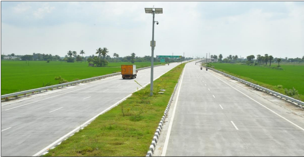
CH: 10+300 TO 11+000 BHS MCW MBCB FIXED IN HIGH EMBANKMENT AREA WITH CHUTE DRAIN, MEDIAN PLANTATION, PTZ CAMERA FIXED
