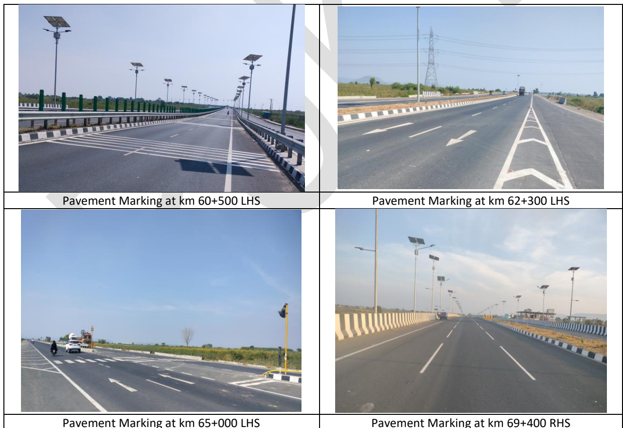
Figure 7.8: Photographs showing the pavement marking Condition
