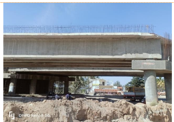
Concrete Crash Barrier pending works at Flyover location
