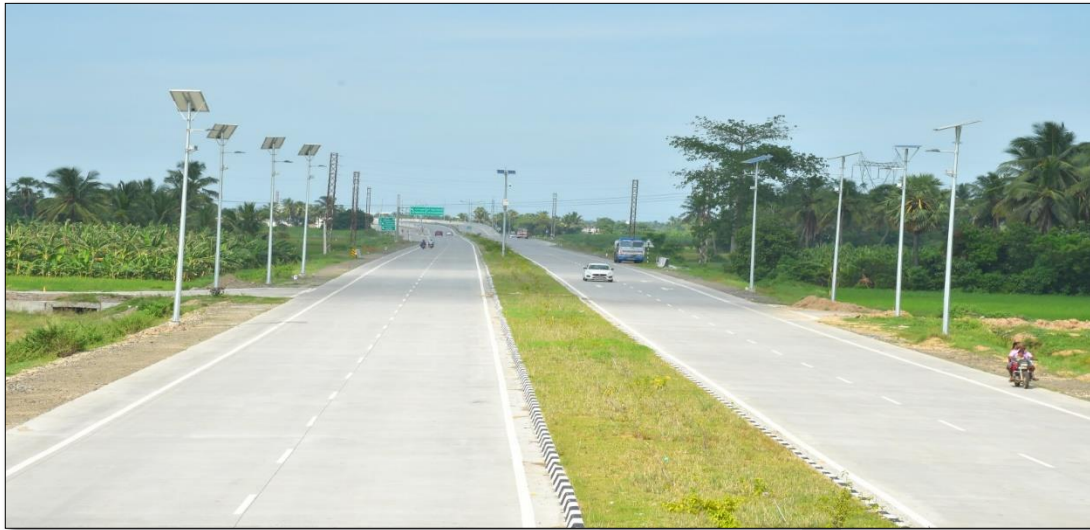
CH: 12+800 BHS MEDIAN PLANTATION, PTZ CAMERA & JUNCTION AREA SOLAR LIGHTS FIXED
