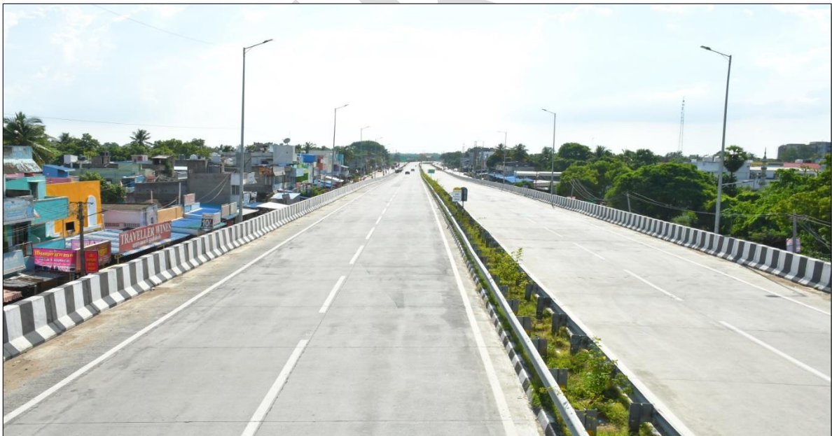
CH: 19+300 TO 20+000 VUP LOCATION MBCB, MEDIAN PLANTATION, RCC DRAIN, URBAN LIGHTS FIXED & SERVICE ROAD WITH JUNCTION
