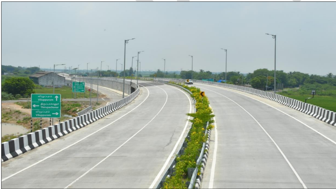
Ch: 3+100 to 3+700 VUP location MBCB, median plantation, Bus shelter, urban lights fixed & Service Road with junction
