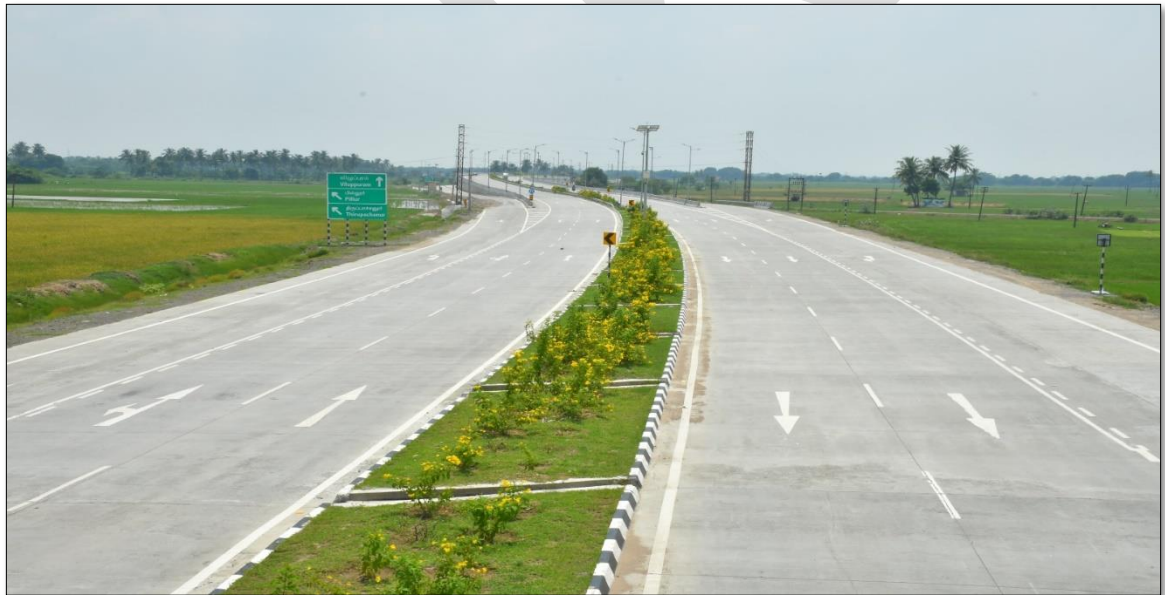
CH: 6+800 TO 7+100 MCW & SR MERGING PORTION, CURVED AREA LOCATION MBCB, MEDIAN PLANTATION, PTZ CAMERA & URBAN LIGHTS FIXED
