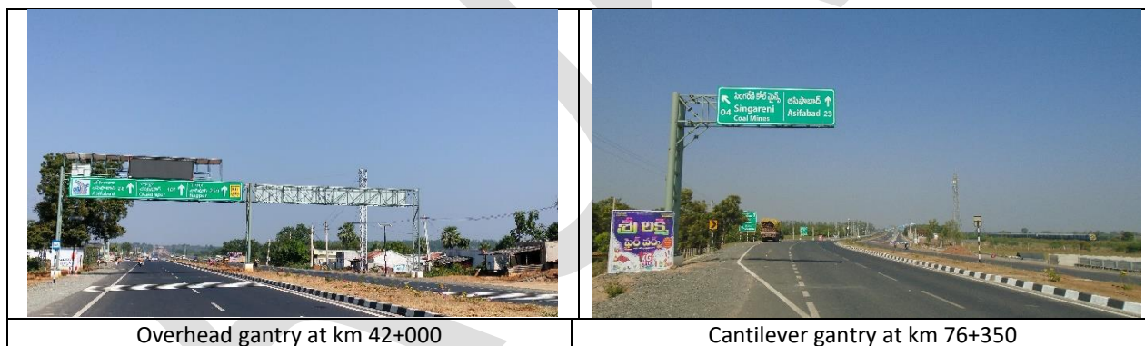
Figure 7.6: Photographs showing the Condition of Overhead sign and Cantilever sign boards
