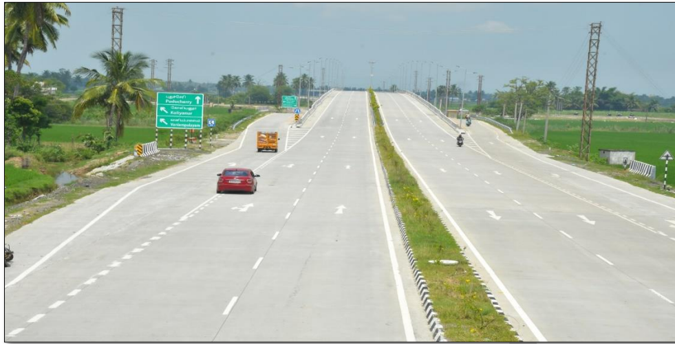
CH: 9+100 TO 9+700 MCW & SR MERGING PORTION, MBCB FIXED IN HIGH EMBANKMENT AREA, MEDIAN PLANTATION, PTZ CAMERA & URBAN LIGHTS FIXED
