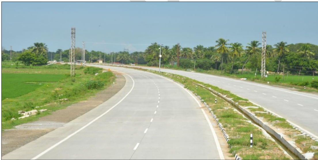
CH: 11+200 TO 12+000 MCW CURVED PORTION, MEDIAN DRAIN, PTZ CAMERA, BUS BAY WITH SHULTER & URBAN LIGHTS FIXED
