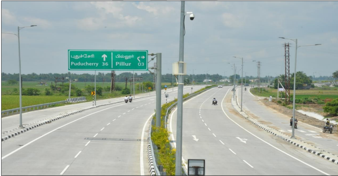
CH: 5+500 TO 6+000 MCW & SR CURVE LOCATION MBCB, MEDIAN PLANTATION, GANTRY BOARD, PTZ CAMERA & URBAN LIGHTS FIXED
