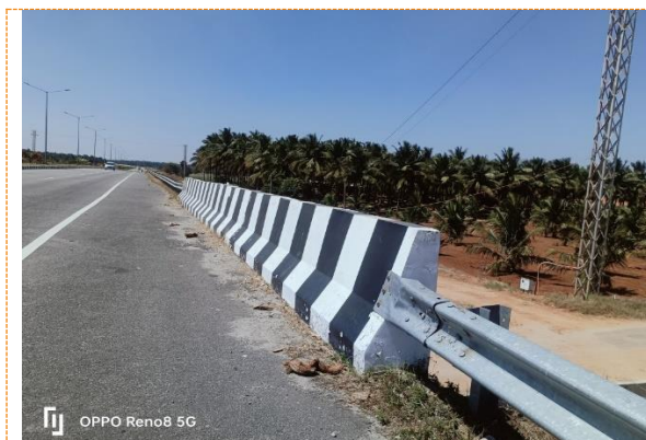
Concrete Crash Barrier @ SVUP location
