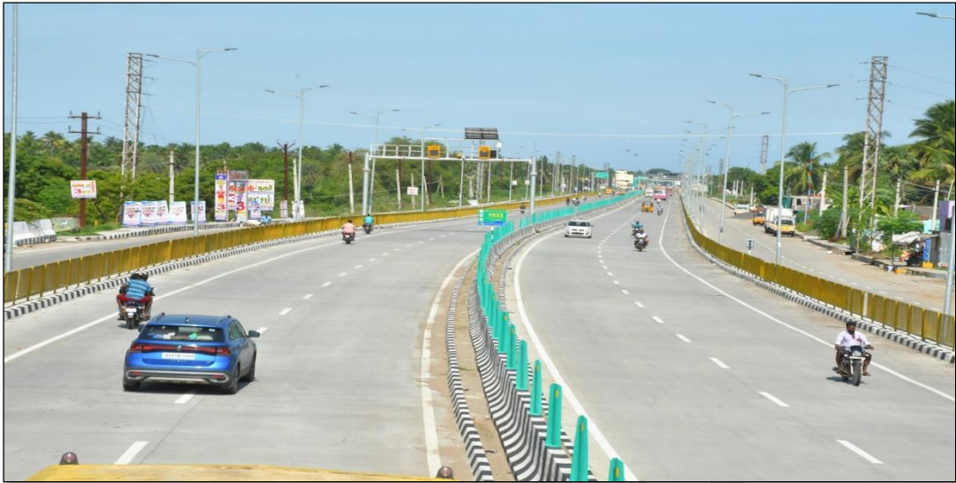
CH: 16+800 TO 17+600 MCW & SR NJCB WITH ANTI GLARED POST, GUARD RAIL, VASD, RCC DRAIN & URBAN LIGHTS FIXED
